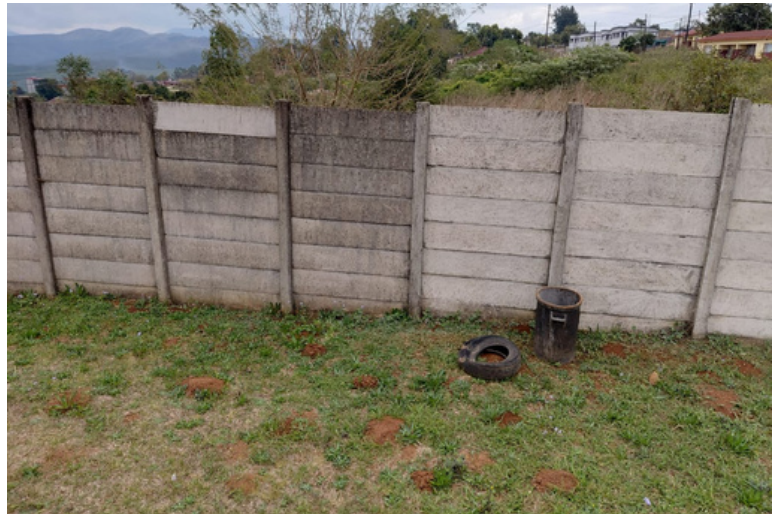
Killarney Sport Ground Scrapped wall vs wall before scraping
