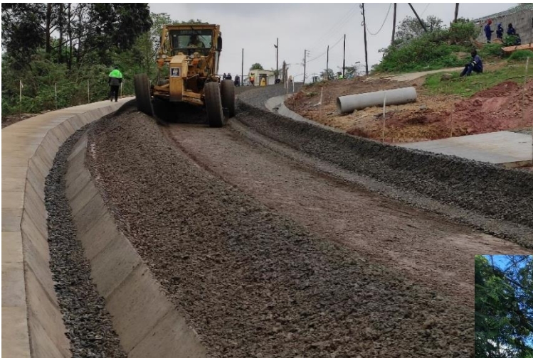
STABILIZATION PREPARATION ON ROAD 1
