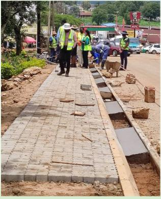
Figure 2.2: Paving of pedestrian walkways
