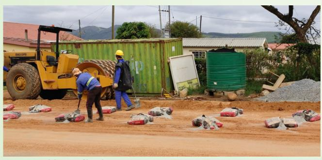
Figure 2.0: Stabilization of base layer
