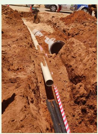
Figure 2.1: Provision of new sleeves for EEC and EWSC
